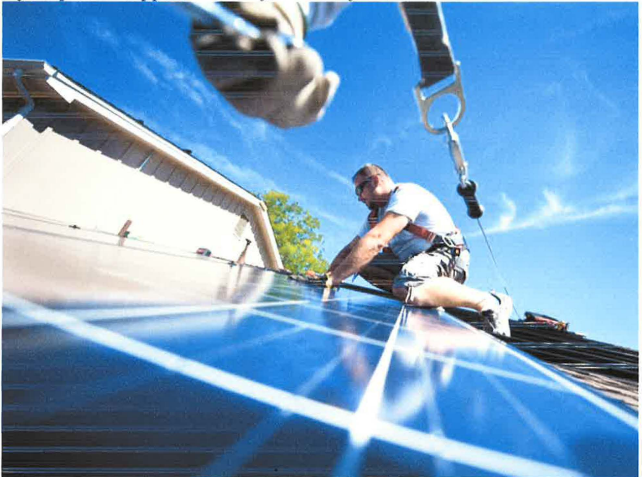
Workers install rooftop solar panels on a home in Colorado.
