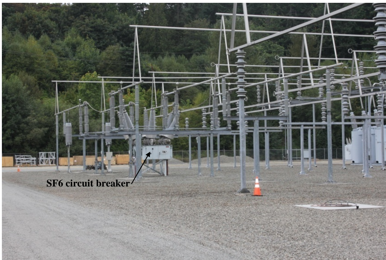
Figure 35. SF6 Circuit Breaker at Sammamish Substation
