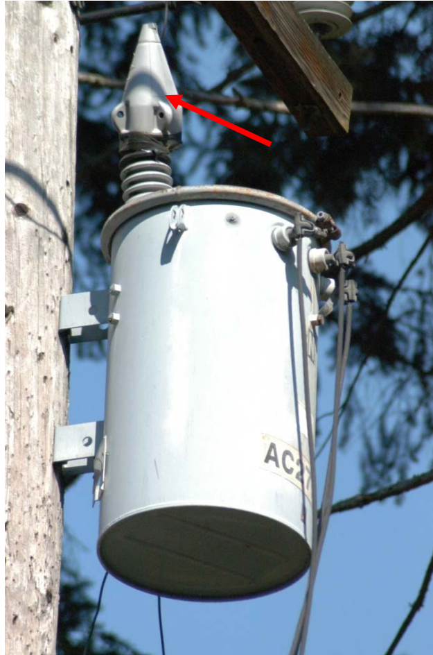
Figure 47. Use of an animal guard (arrow) to prevent inadvertent contact at the top of an overhead service transformer
