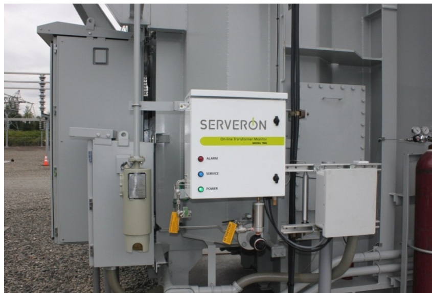
Figure 39. Transformer equipped with a modern on-line gas-in-oil monitor at Sammamish Substation
