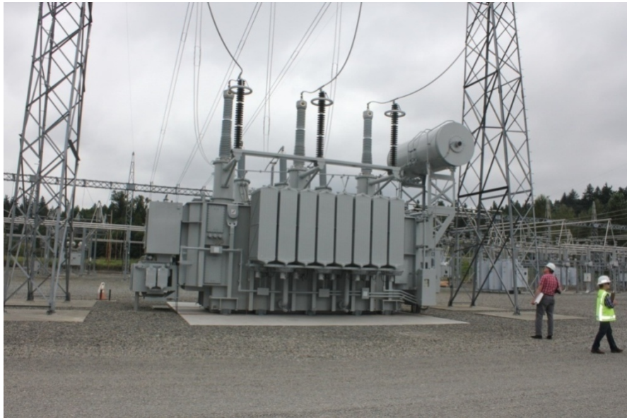
Figure 38. New 325 MVA Transformer at Sammamish Substation
