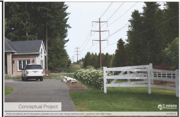
Above: Photo simulation representing double-circuit monopole structure in Bridle Trails (Bellevue).
